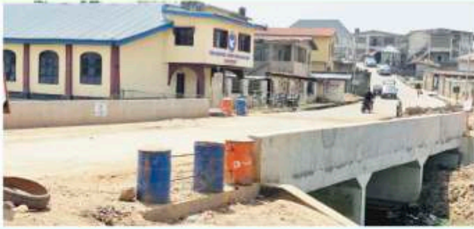
ID 633 (3-Cell Culvert on the Orogun River by GOFAMINT Church)
