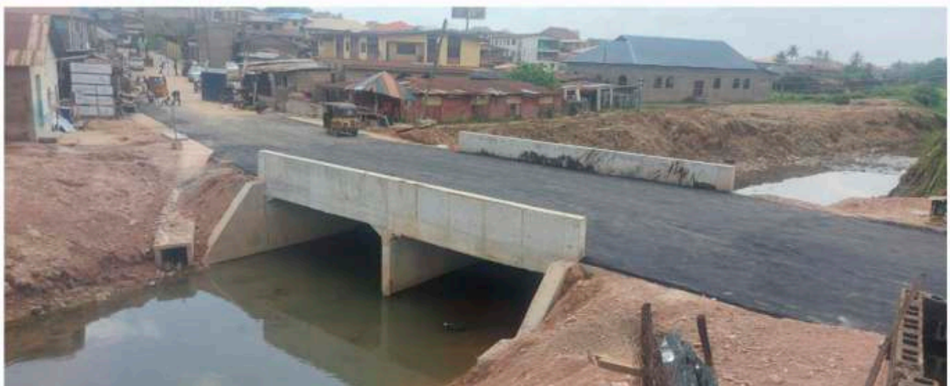
Culvert G5 at Akinwumi-Odewenwa Street off Iwo Road
